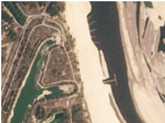
ZNPP water intake channel showing pipelines in Kakhovka. Reservoir, July 25, 2023 Source: Planet Lab
