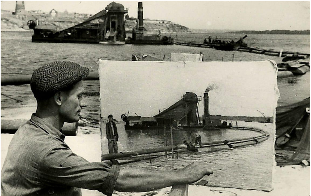
Ukrainian artist Albin Havdzynskyi working on one of his paintings dedicated to the construction of the Kakhovka HPP. Source: Istorychna Pravda 8
