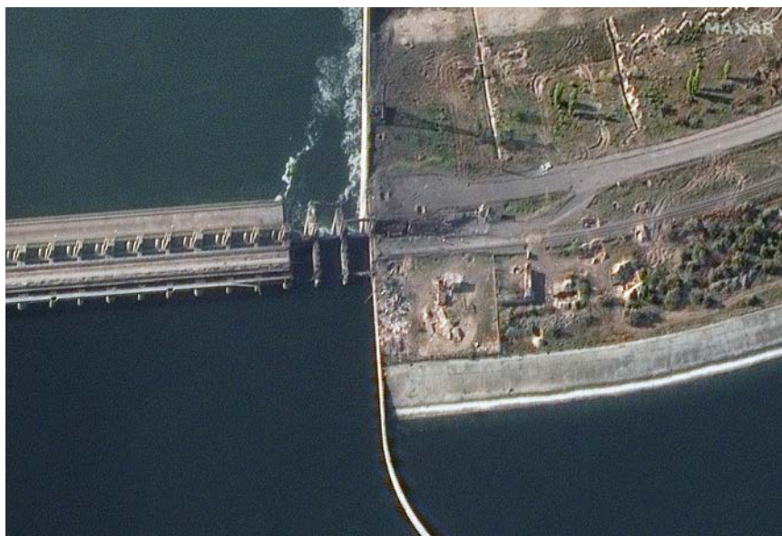
Satellite image of the damaged 3 spans by the Russian military Source: Maxar, November 11, 2022 773
