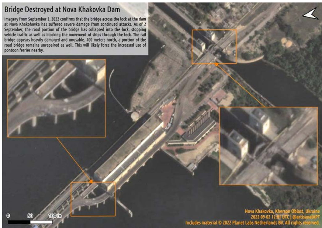
Satellite imagery of the destroyed bridges. Planet imagery from September 2, 2022. Source: @mil.in.ua
