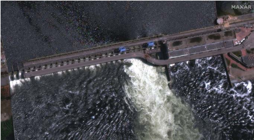
Kakhovka Dam on May 28, 2023. Source: @evanhill via X
